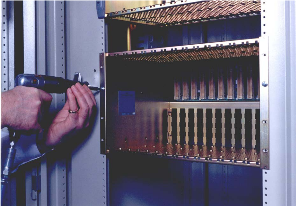
Figure 9 Installation of Chassis
