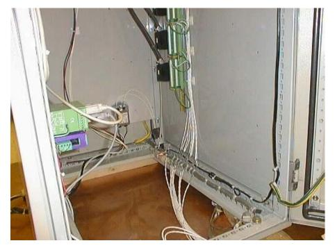
Figure 9-5—Bottom Cable Entry Area
